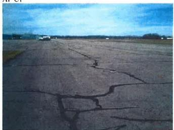
AP C2 & D: No preventative maintenance has been done on this pavement. Crack seal and seal coat.
