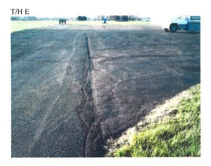
T/H F: Seal coat pavement is starting to ravel.
