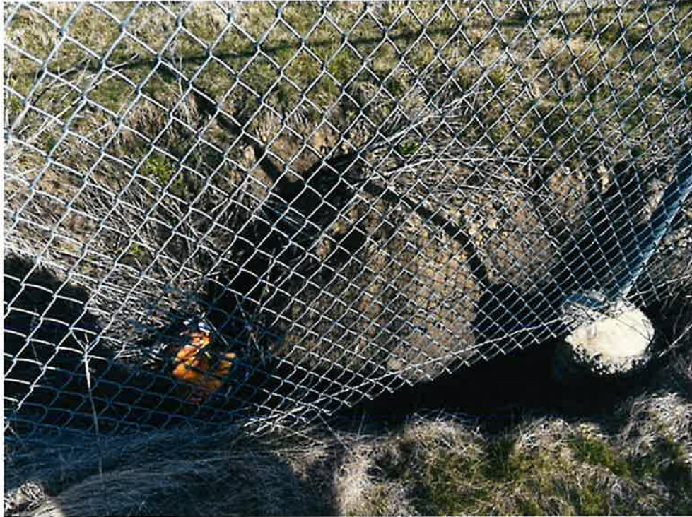
Picture 2: Blowhole erosion (site by 11)
