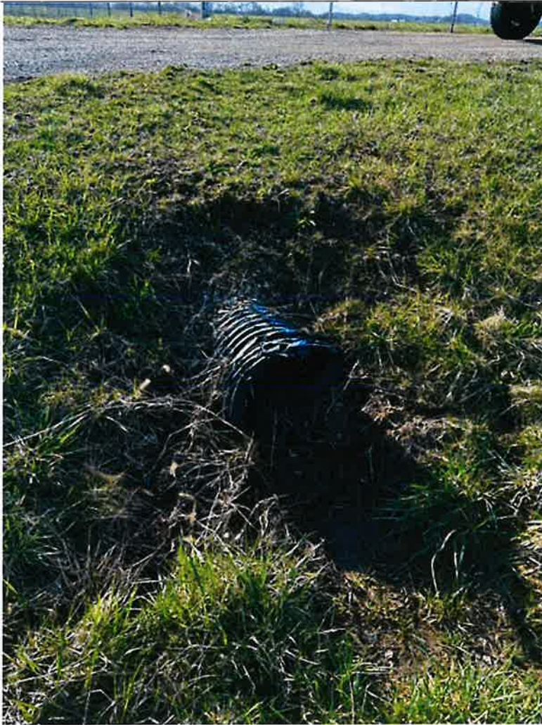
Picture 1: Damaged culvert (site 12) ARF Road
