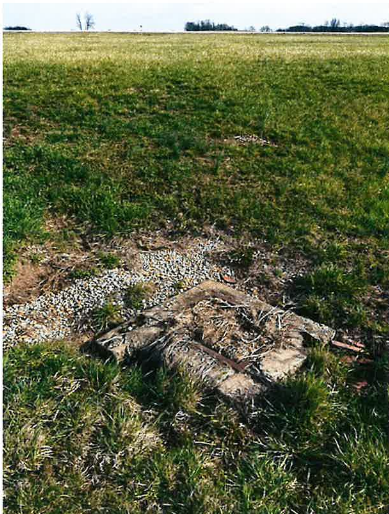
Picture 5: Drain was blocked by grass, in infield location. FSWCD removed buildup.
