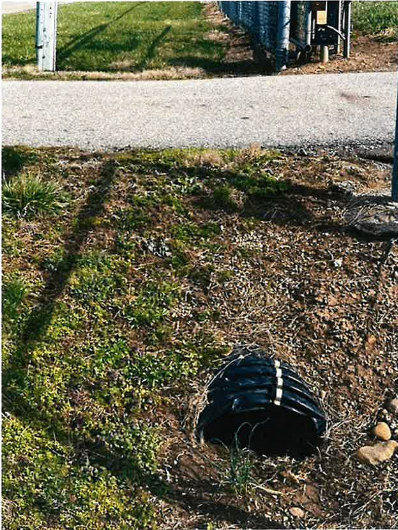
Picture 4: Culvert needs dipped (site 3). East gate to hangars.
