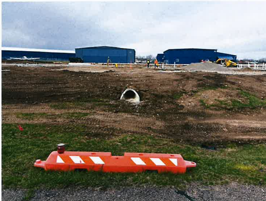
Picture 9: Where drainage pipe exits needs wattles or silt fencing around un-stabilized soil.
