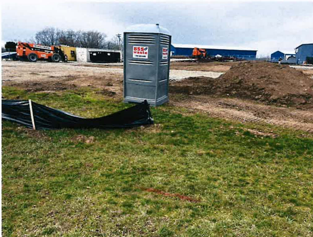
Picture 7: Slit fencing needs repaired or replaced and extended.
