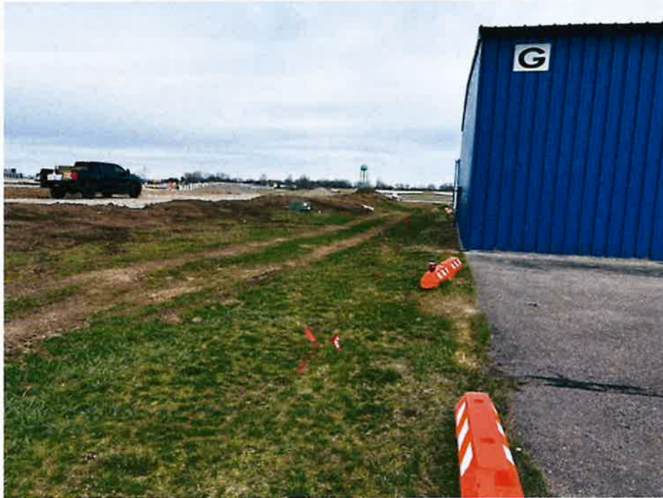
Picture 8: Area needs silt fencing or wattles around un-stabilized soil.
