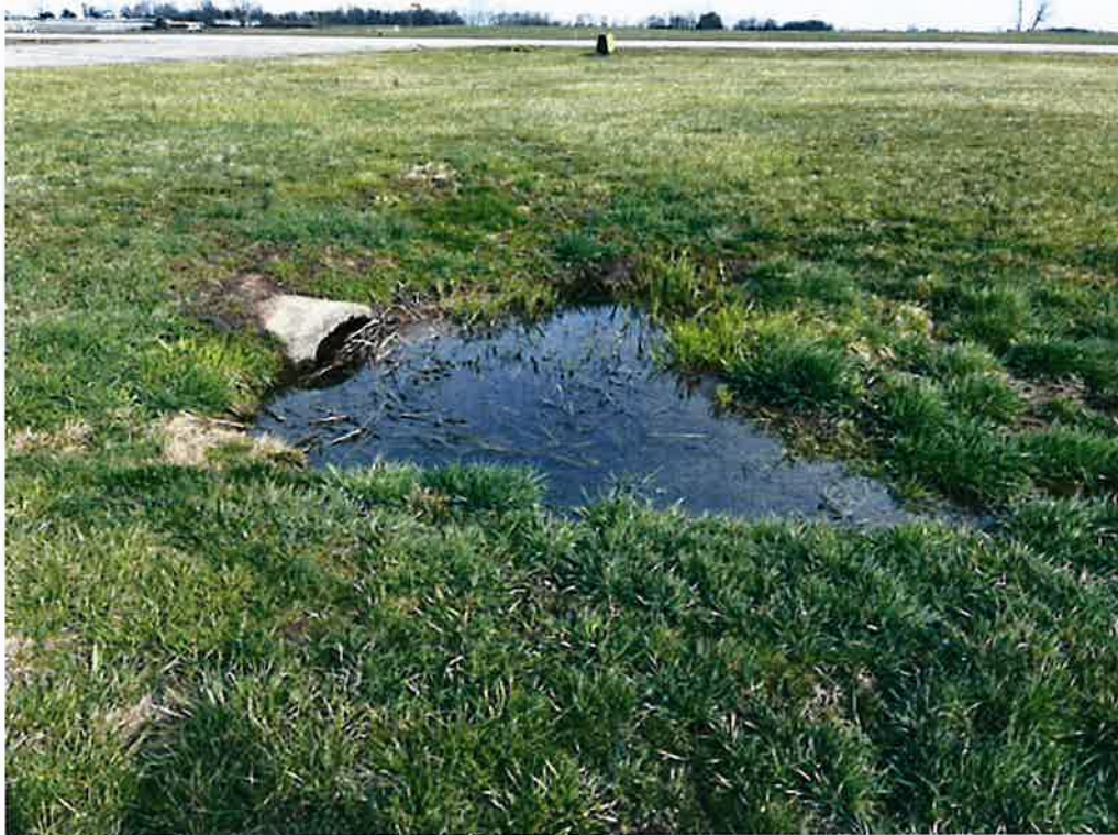
Picture 6: Culvert where the tile meets the drain needs repaired. (infield)
