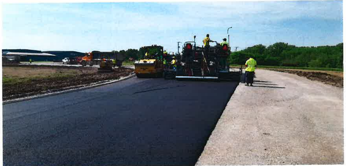
Asphalt Paving has started
