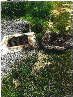
System #7 Ditching and drainage improvements made last year are still providing positive flow and reduced ponding in the infield. It is assumed there is a spring flow in the infield providing the constant source of water.
