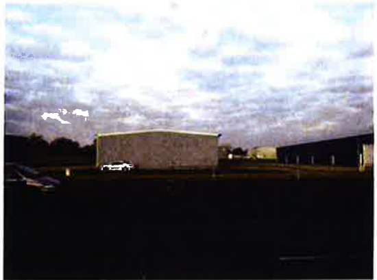
FP 1: Looking west.
