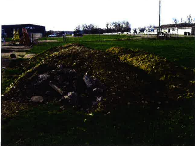
Figure 10. Dirt pile near cement pads and apron.
