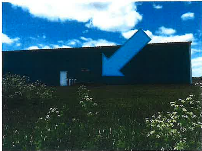
Blue barrel stored outside Hanger R -East side should be reviewed by Board
