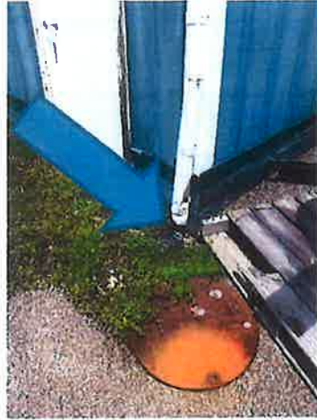
Building J downspout disconnection
