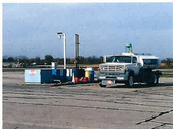
Fuel Farm and Fuel Truck (10-31-16)
