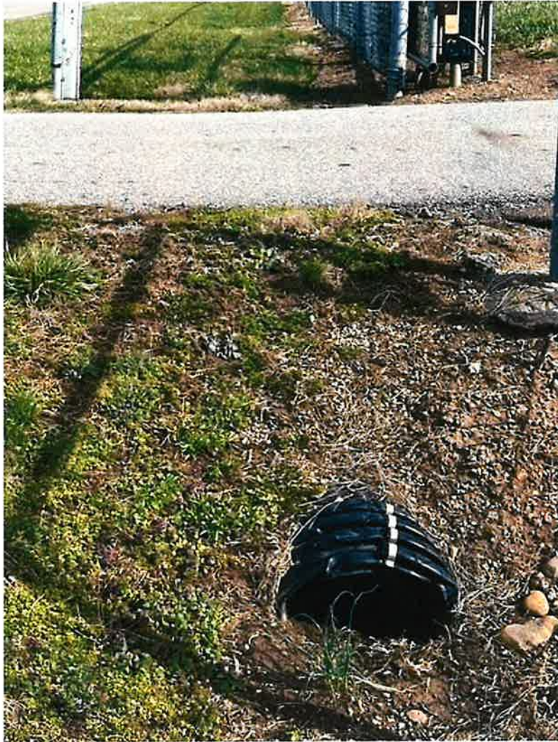
Picture 3: Culvert needs dipped (site 3). East gate to hangars.
