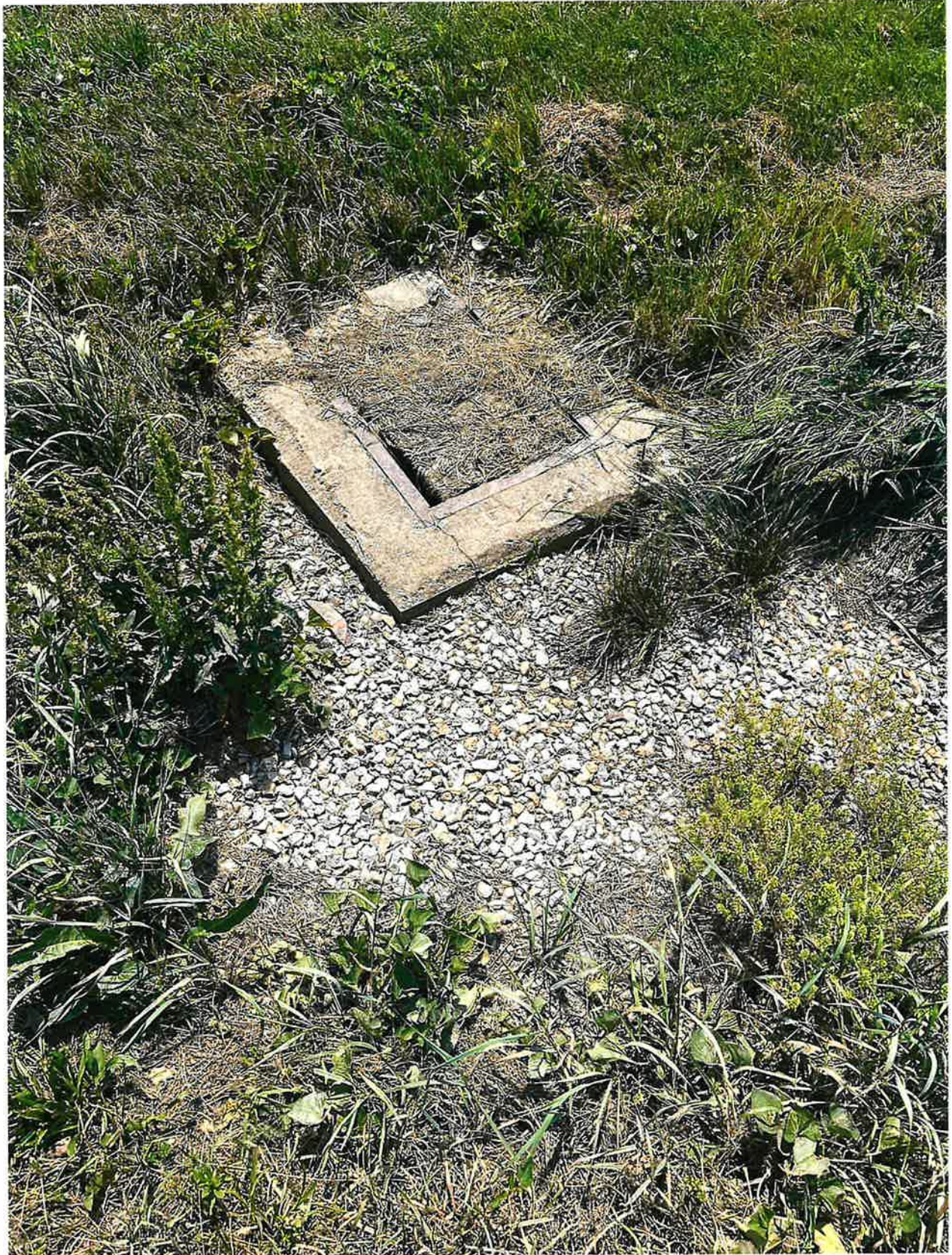
Picture 4: Drain was blocked by grass, in infield location.
