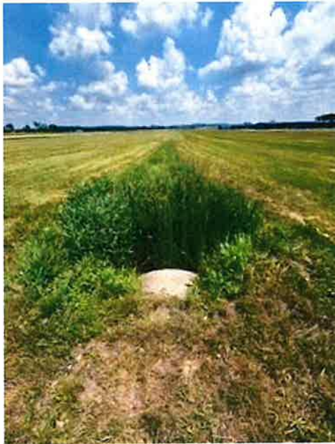
Picture 5: Culvert where the tile meets the drain needs maintained. (infield)
