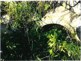
System #4 NW Corner of Building R, edge of pavement erosion. Reinforce/fill with rip-rap.
