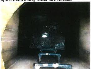
System #3 Outfall of pipe passing under build Q is filling with sediment. Source not observed. Clean and monitor.
