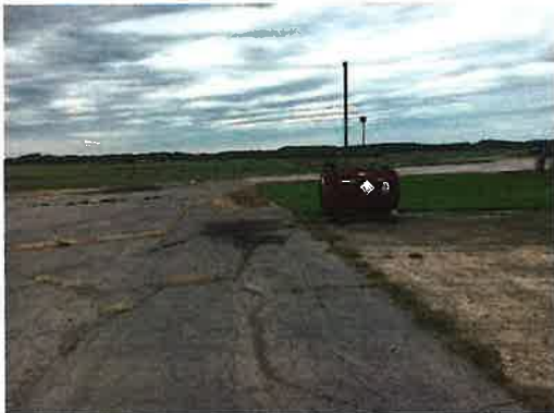
Diesel spill west gate
