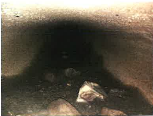
System #2 gravel build-up at offsite release
