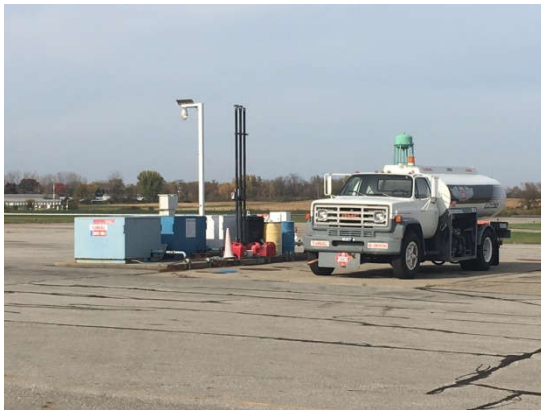
Fuel Farm and Fuel Truck (10-31-16)
